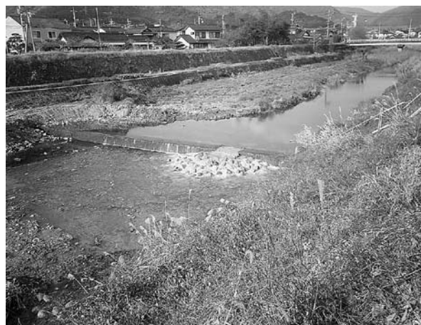
Fig. 5. “Mizube-no-Kowaza” fishway constructed to the Fushino River.
