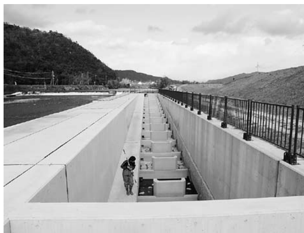
Fig. 2. The conventional type of fishway for large-sized fish such as salmon or trout.
