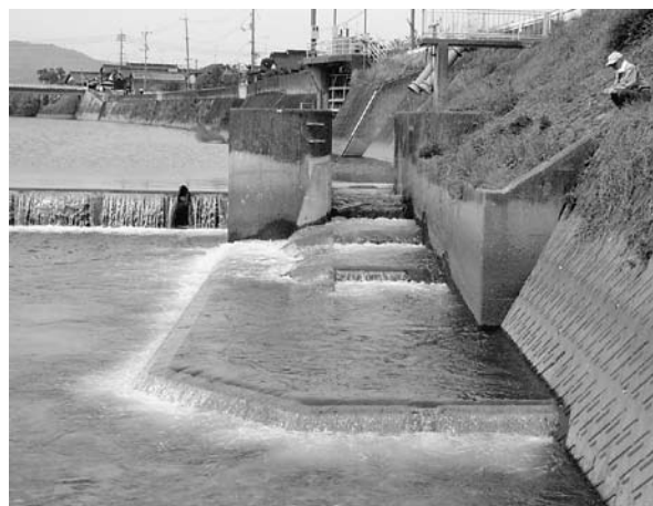
Fig. 10. Improved fishway in the Asa River. Sidewall of fishway was removed.
