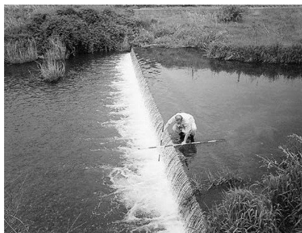
Fig. 4. A weir (drop) at the Fushino River in Yamaguchi Prefecture before the construction of “Mizube-no-Kowaza” fishway.
