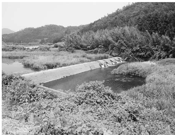
Fig. 6. A small dam (head works) with five sliding timber weirs at the Ooi River in Yamaguchi Prefecture before the construction of "Mizube-no-Kowaza" fishway.
