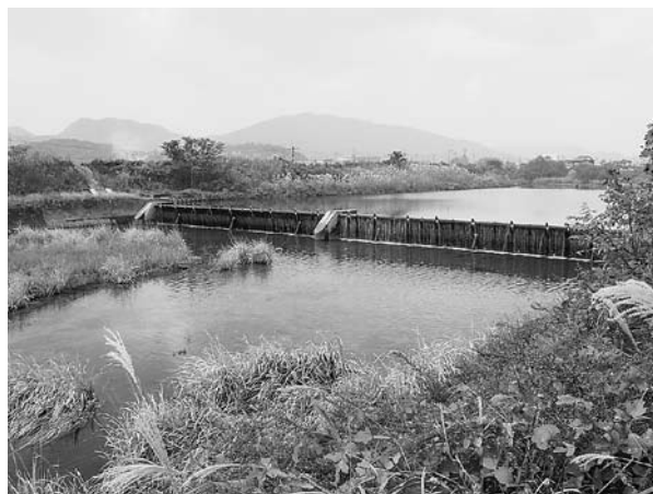
Fig. 1. Many artificial structures like weirs and dams constructed across Japanese rivers prevent the migration of aquatics.
