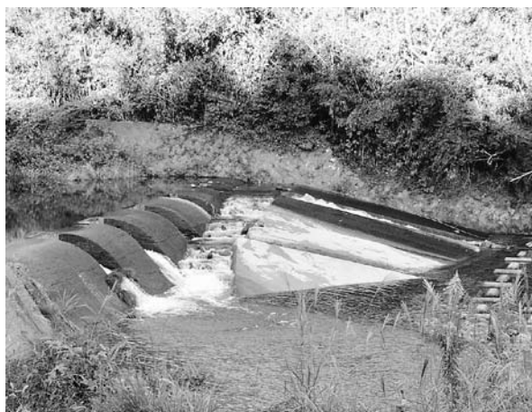
Fig. 8. "Mizube-no-Kowaza" fishway constructed the Ooi River.
