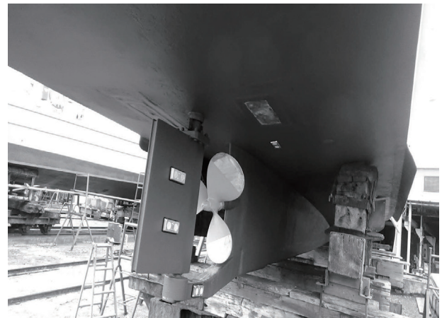
Photo3-2 Condition of rudder and propeller after cleaning
