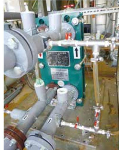
Fig.3 Test heat exchanger (Plate type)
